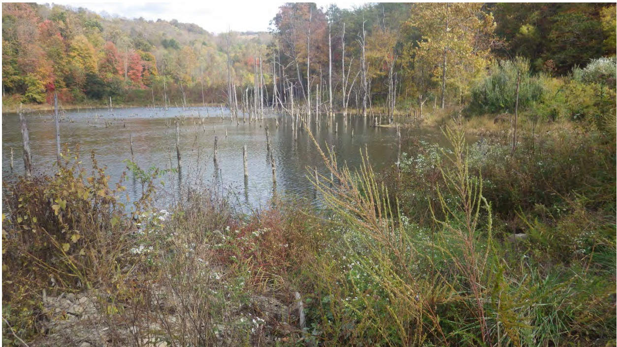
Photo 114 – Reach 8 – overview of pond
