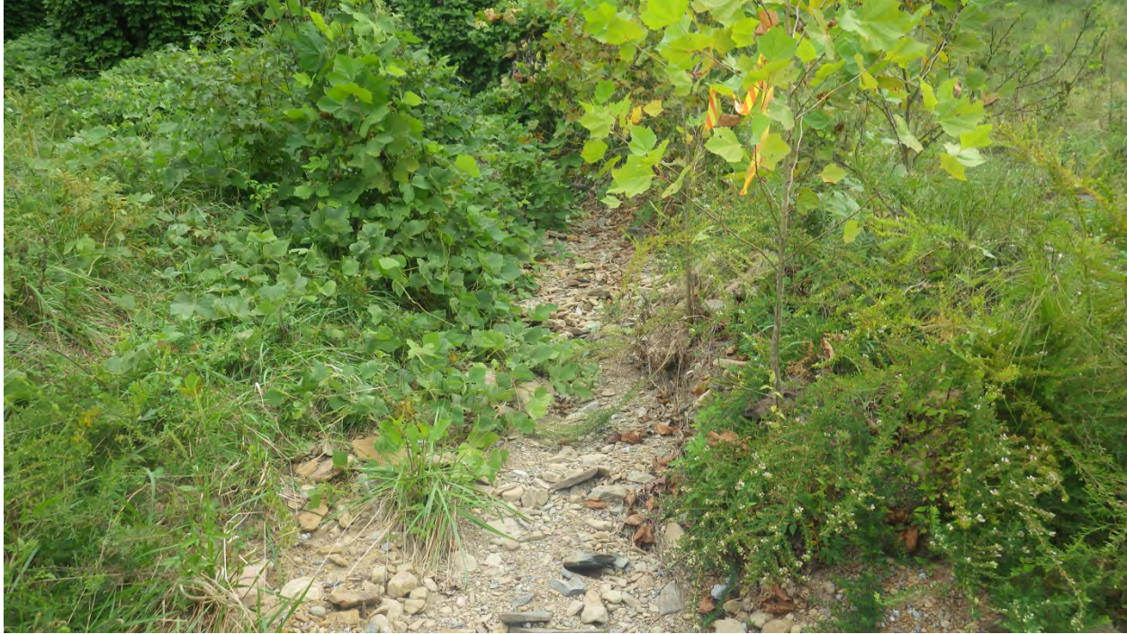
Photo 1374 – Old Hollow Fill side drain facing upstream
