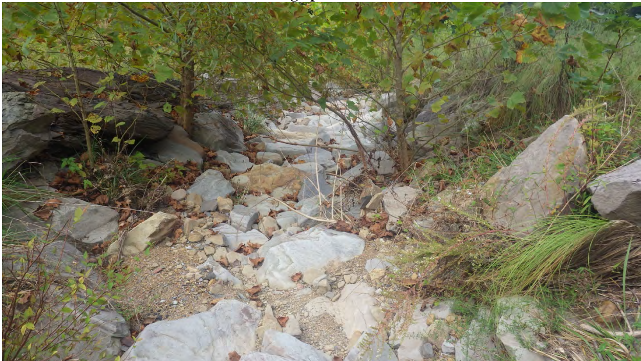
Photo 1375 – Old Hollow Fill side drain – facing downstream
