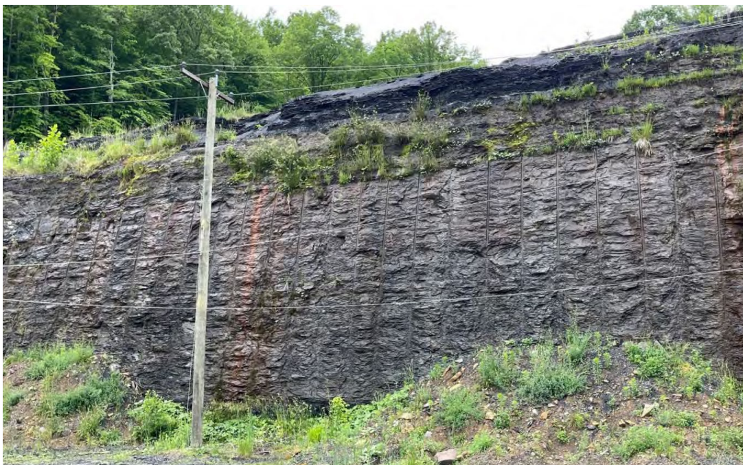
Figure 5-32: Closed High Wall Mining Operation in Project Vicinity
